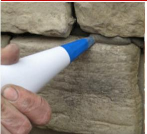
**U-POINT** is a single component, polymer modified, water resistant, cement based compound used to repoint all types of masonry joints.
