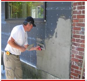
U-TROWEL BASECOAT is a blend of Portland cement, select aggregates & alkaline resistant fibers designed to be used as a basecoat for U-Trowel, Finish-Coat, manufactured stone and thin stone veneers.
